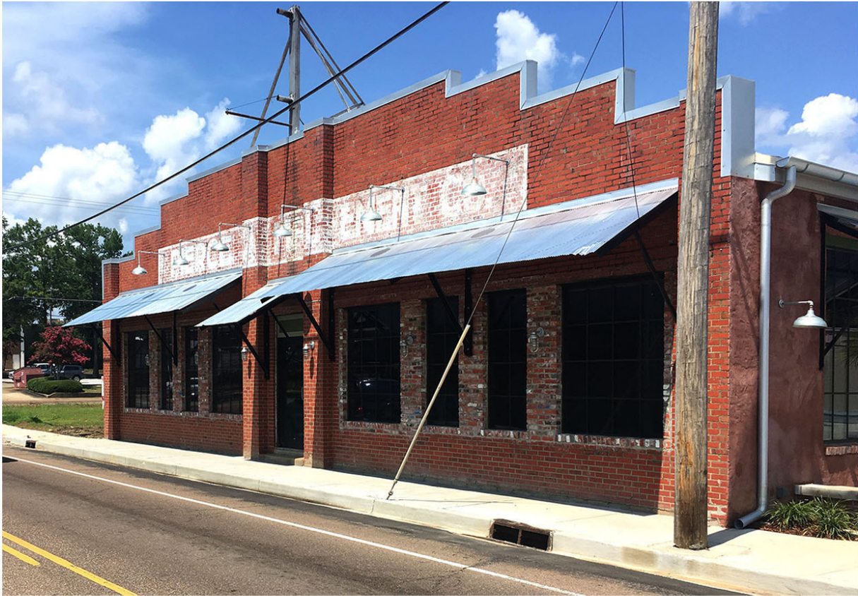
Jackson Square _ Hewlett Building _ 210 Jackson Street _ Parcel 384 _ T5 District
