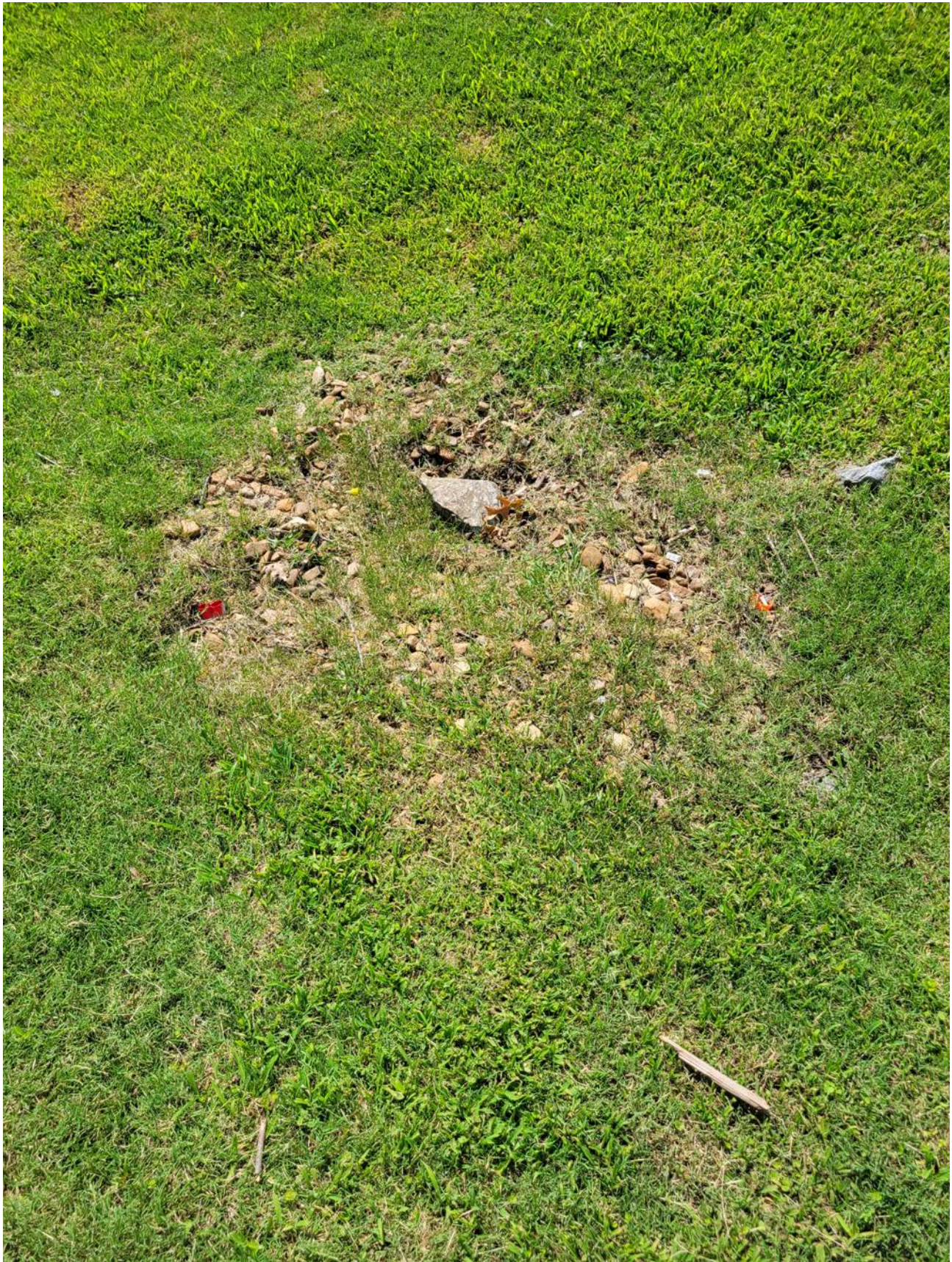
Existing Drainage Structure
