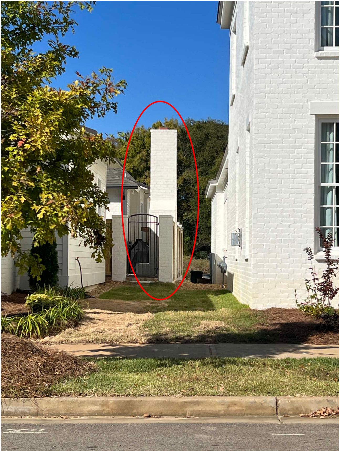
Attachment 3- View of fireplace from street looking north
