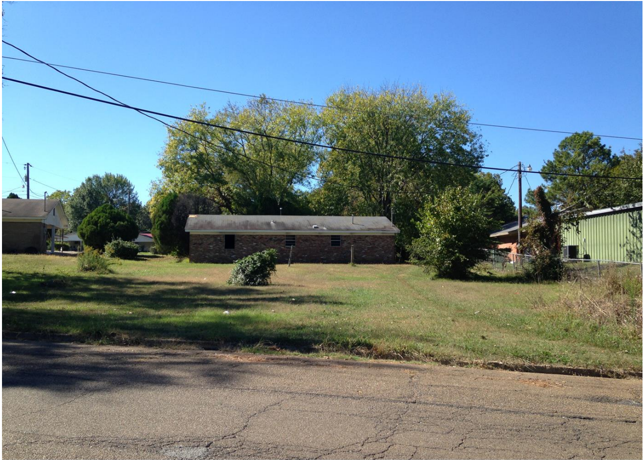
View looking west from North Long Street at the rear of the existing house
