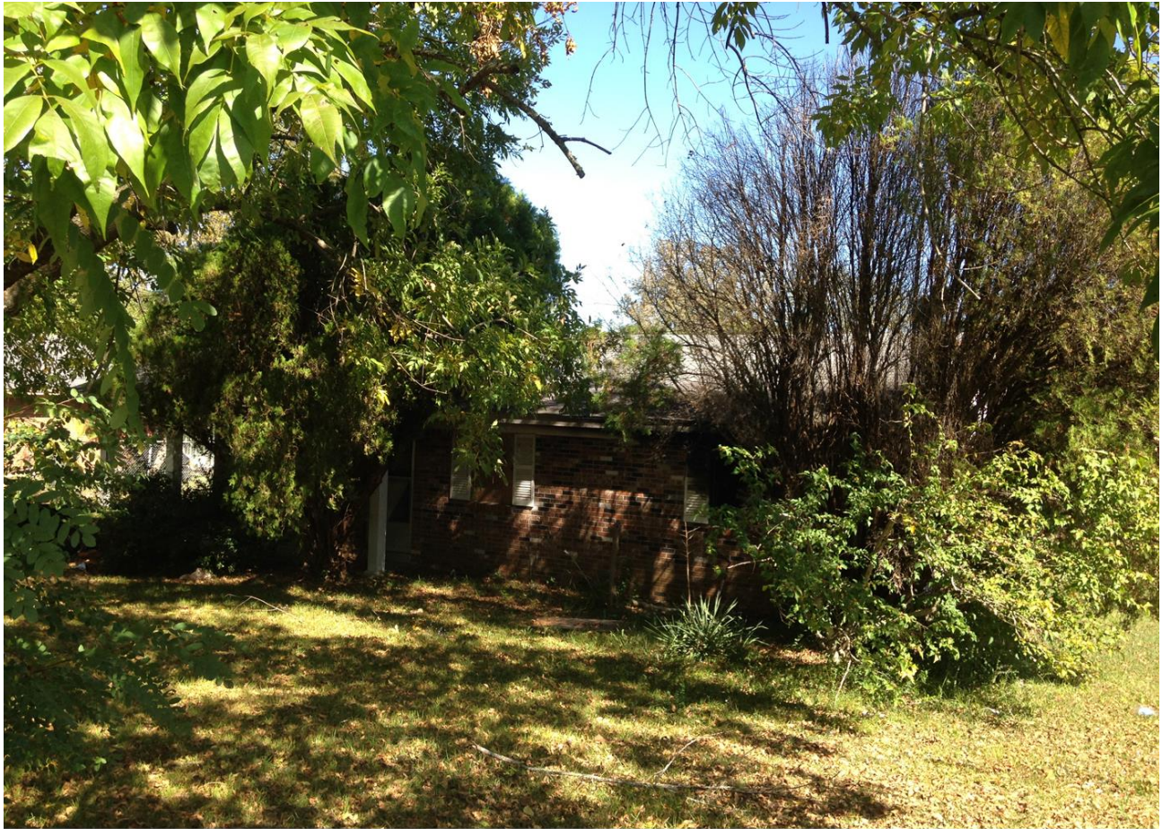
View looking at the front of existing house from Evergreen Avenue
