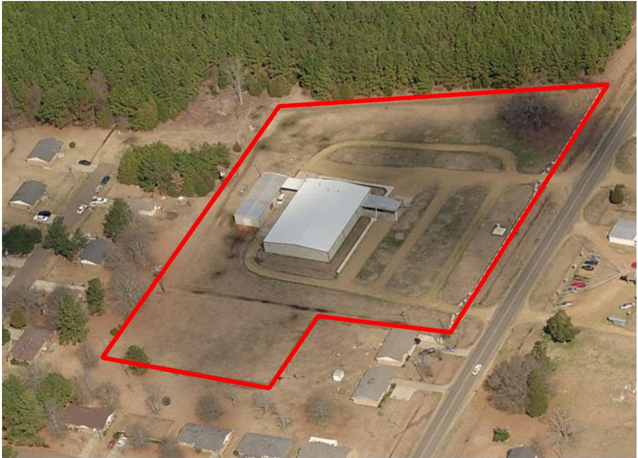
View of subject parcel looking northwest
