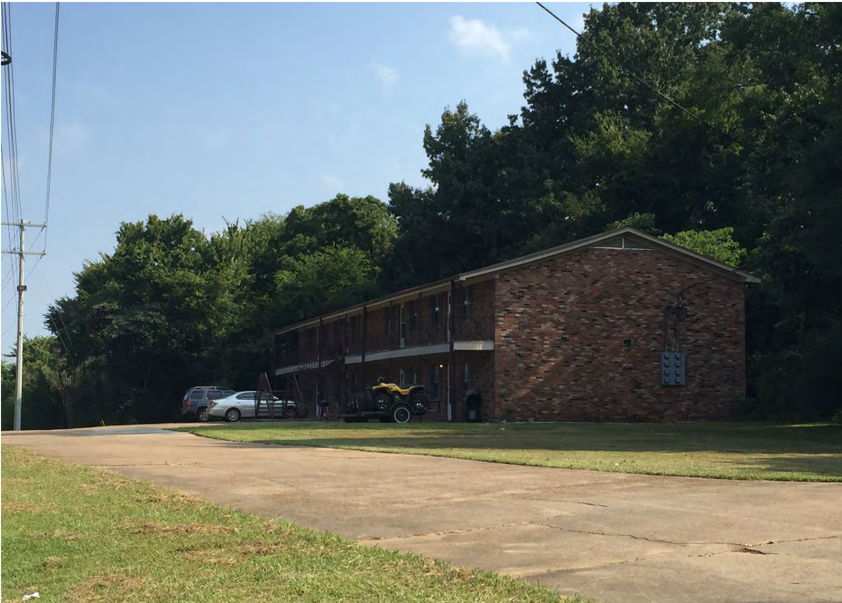
View looking north at existing apartment building on subject properties
