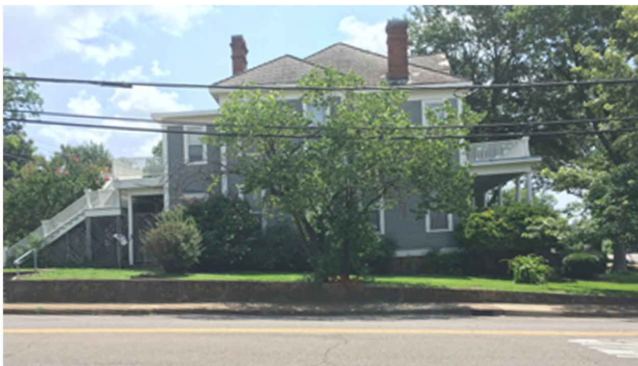
view of subject properties facing West on North Montgomery Street
