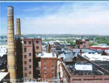
Armstrong Floor Plant, Lancaster, PA
