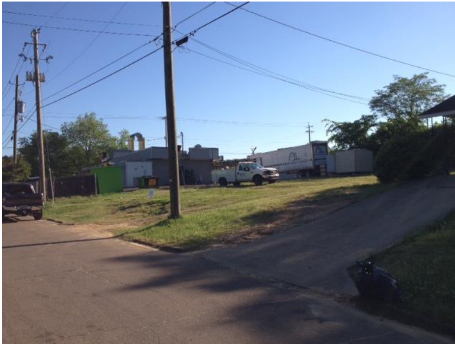
Street View - North
