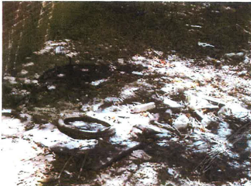
Open cleanout behind building
