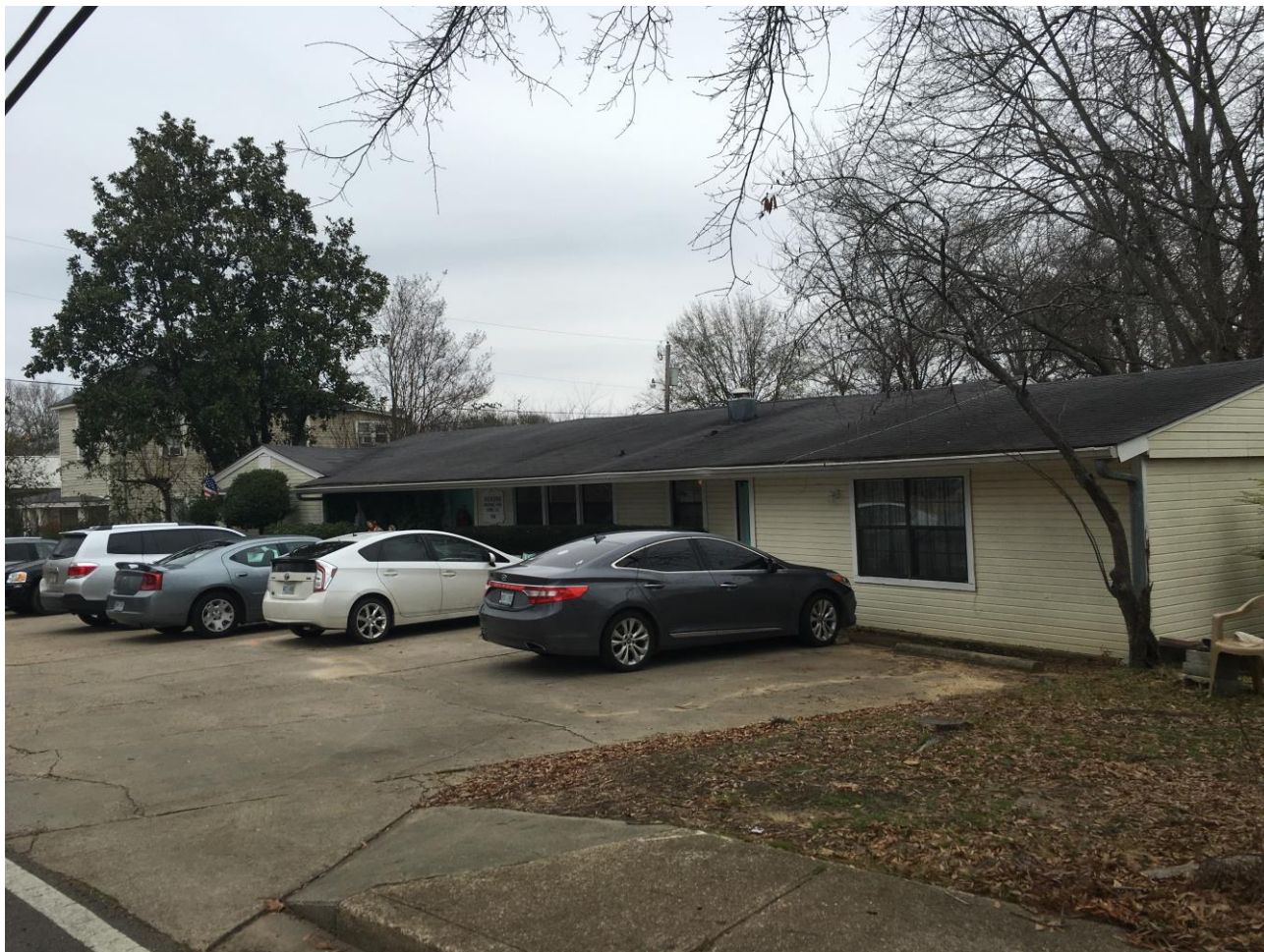
Attachment 3- View from the street of subject property facing east
