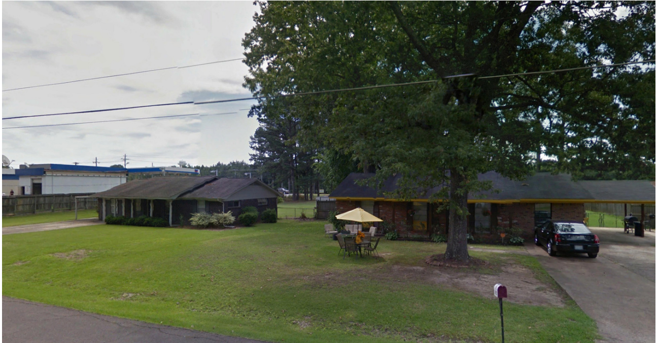
View looking south at front of subject properties
