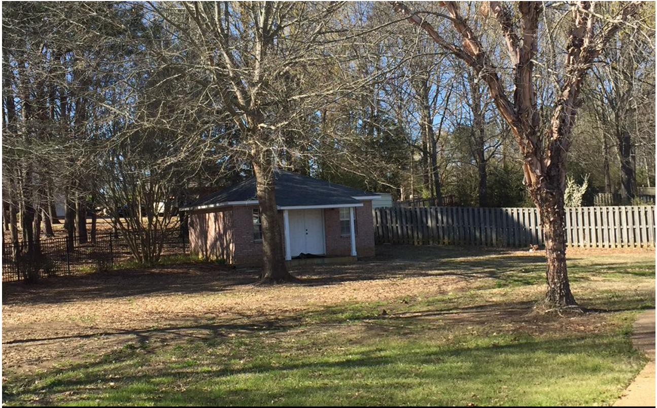
View of existing structure
