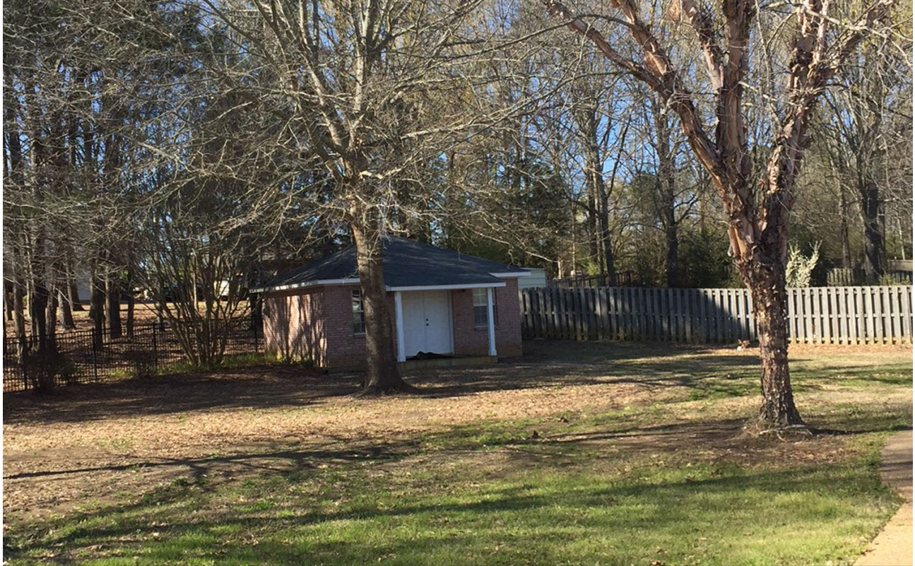
View of existing structure
