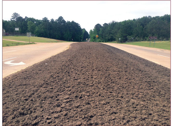
Figure 1. This elevated median was tilled before sowing. Multiple passes over a site may be required to break down large clods. A smooth soil surface prevents broadcast seed from getting buried too deep between clods during weathering.
