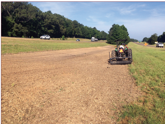
Figure 2. Cultipacking after seeding allows the seed to be pressed into the soil surface, allowing for greater seed-to-soil contact, which enables seed to imbibe water and nutrients for germination and development.
