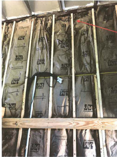
Interior wall view
