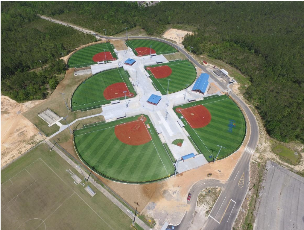
Figure 2: Gulfport Sportsplex Phase III – Synthetic Turf/LED Lighting. Image before bleachers and shade structures. (Picture Drone image Brown Mitchell Alexander (BMA) Engineering)
