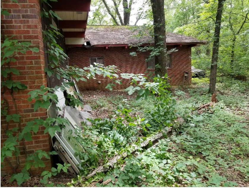
Excessive growth of weeds and other noxious plants on the land
