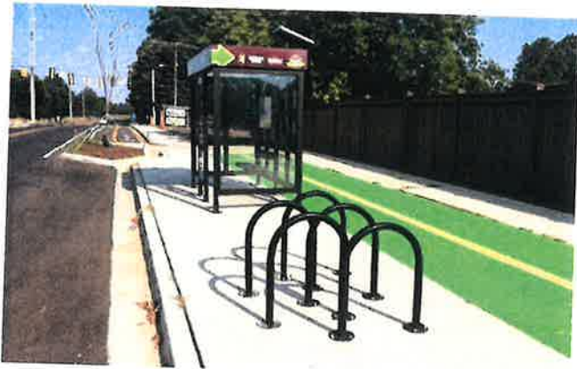
Multimodal stop installation on Locksley Way in Starkville, MS
