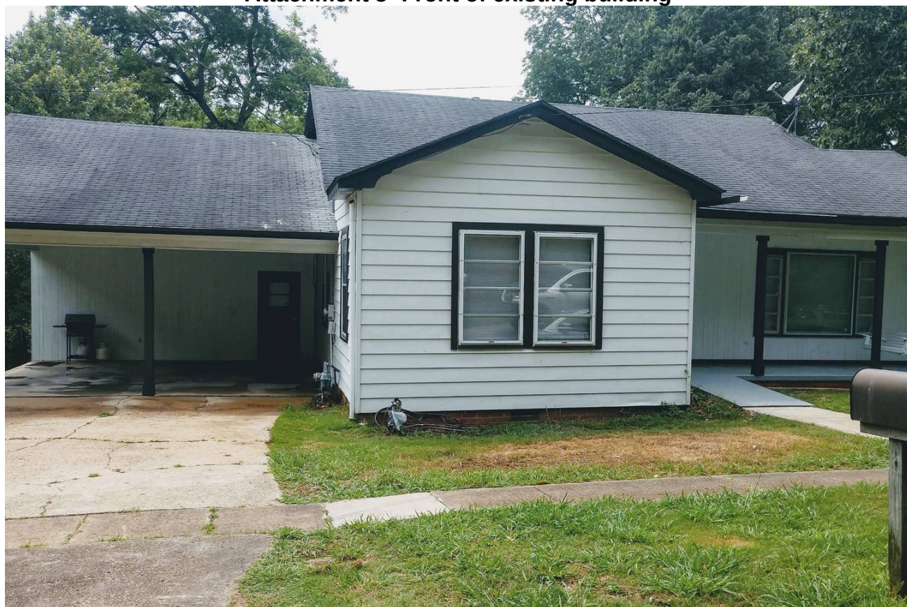
Attachment 3- Front of existing building
