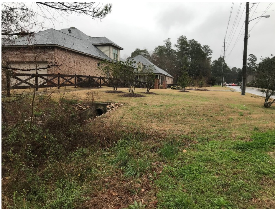
Photo Location 2 – Looking east at drainage pipe within ROW at Riddle Run's southwest corner.
