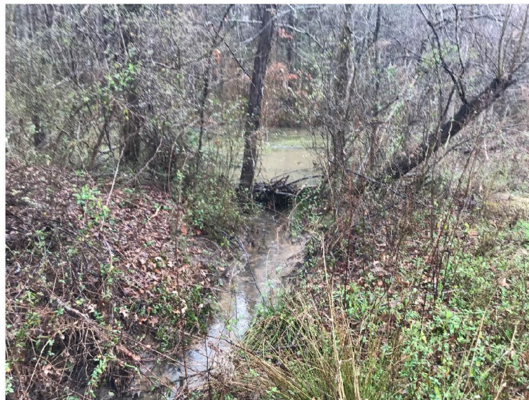
Photo Location 13 – Outlet of shallow pond flowing towards culvert under Lynn Lane.
