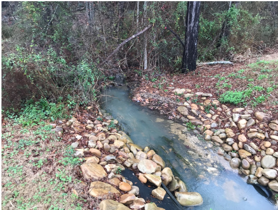
Photo Location 2 – Flow from drainage pipe discharging within ROW at Riddle Run's southwest corner into a swale through Richmond Property.
