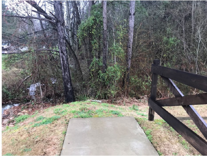
Photo Location 1 – Looking west at western end of sidewalk/fence at Riddle Run.
