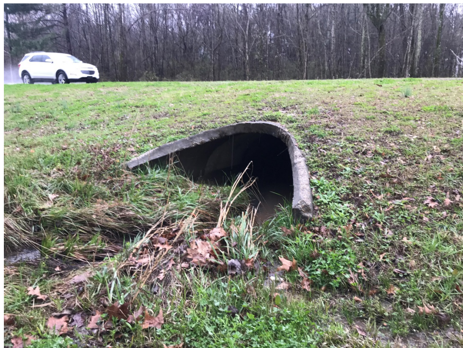
Photo Location 14 – Close up of culvert catching roadside swales from the east and west of this low point and conveying water under Lynn Lane to ditch that flows to the south.
