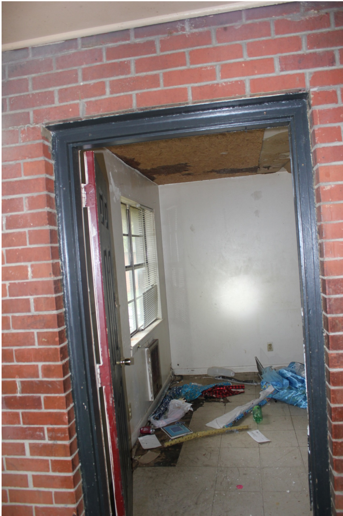
Building # 5 Apartment C Entry way
