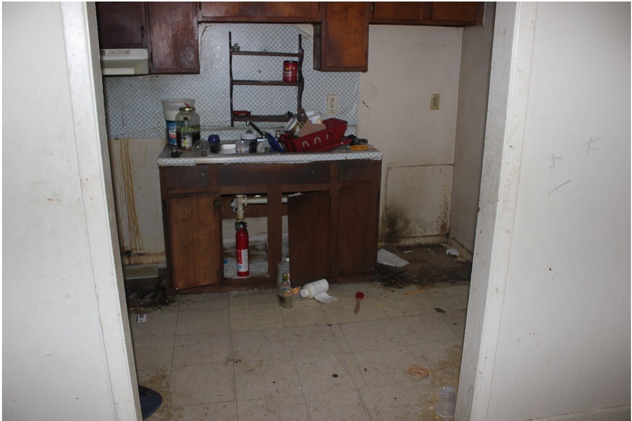
Fire extinguisher 9 months out of date.
