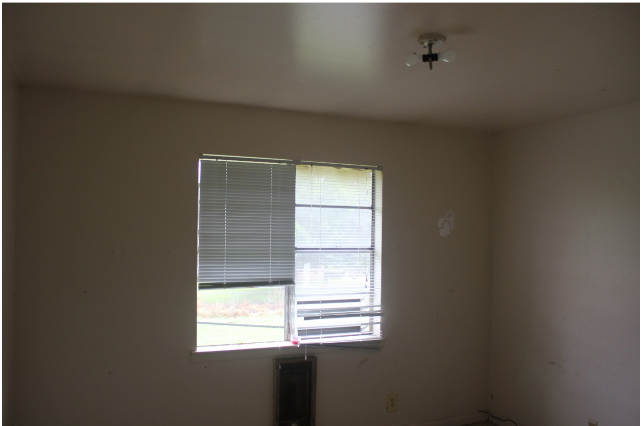
Window not secure and outdated heating unit.
