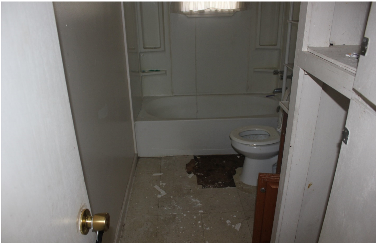
Bathroom floor tiles missing and soft floor from water damage.
