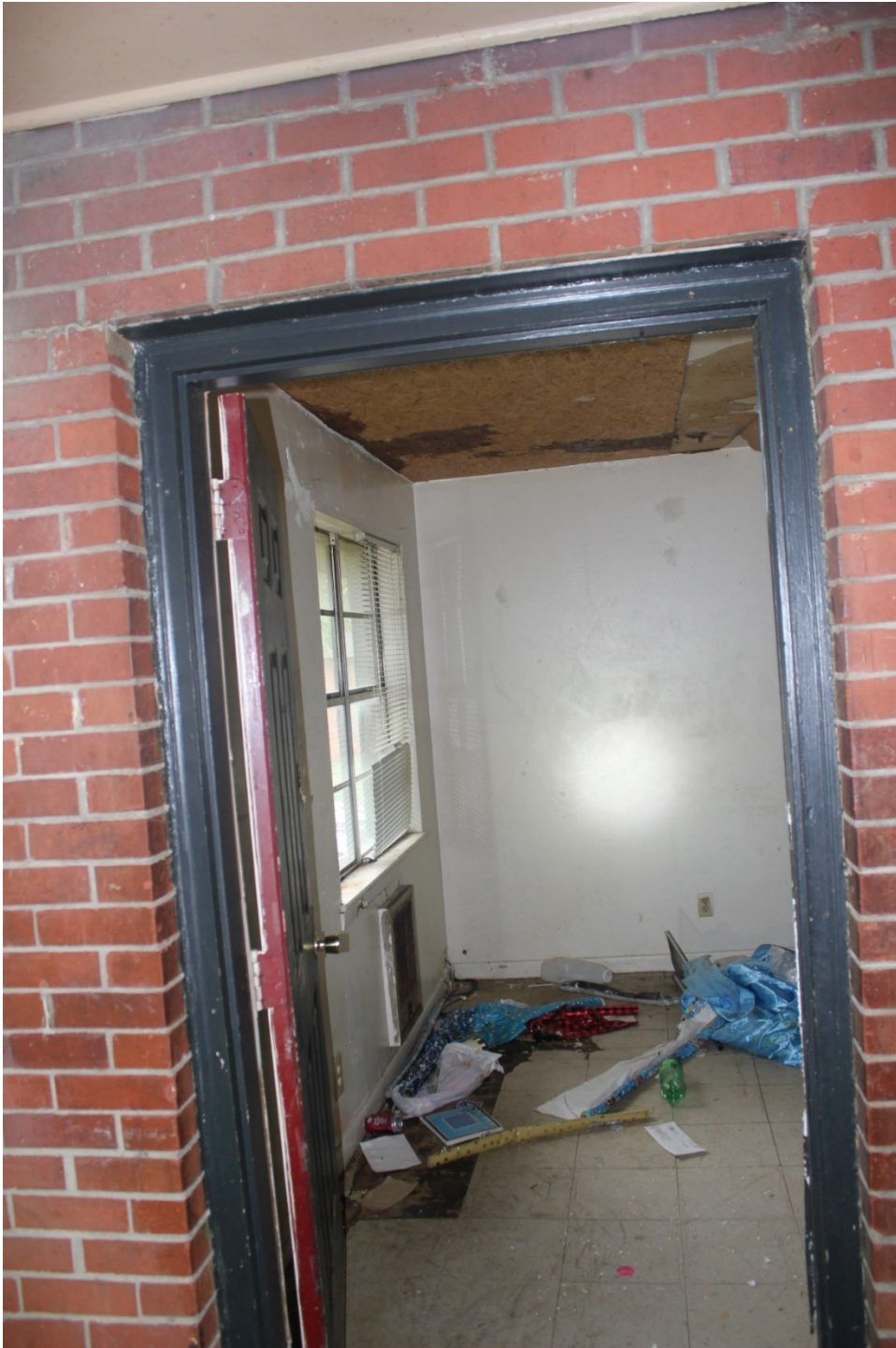
Building # 5 Apartment C Entry way
