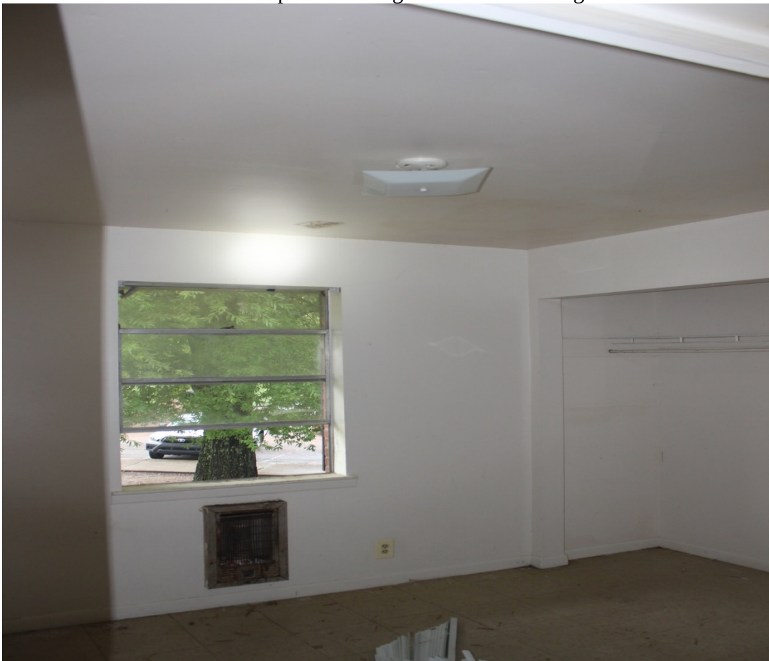
Discolored spots in ceiling - Outdated heating unit - Unsecured window
