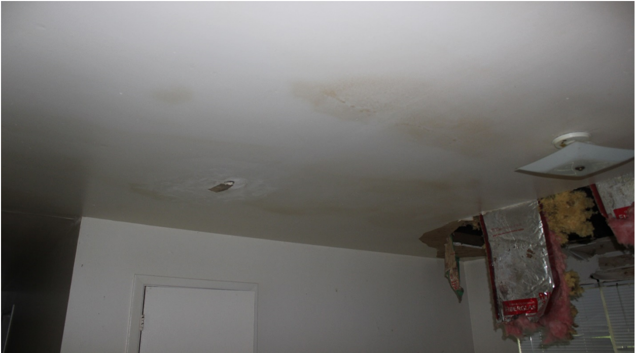
Discolored spots in ceiling - Outdated heating unit - Unsecured window
