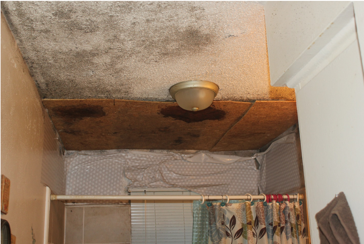
Bathroom hole in ceiling covered by a piece of plywood and mold growth across the ceiling and making its way down the walls.
