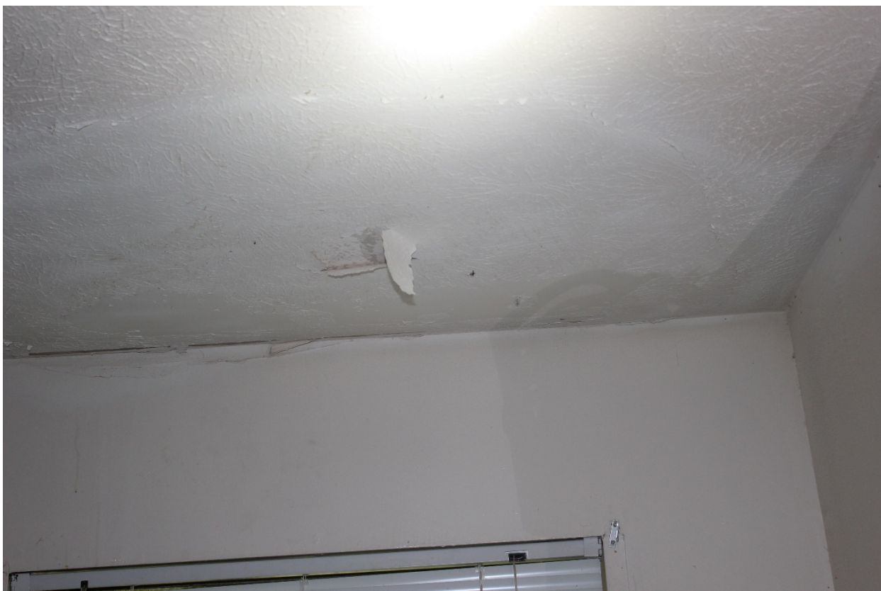
Kitchen ceiling is beginning to show signs of water damage.
