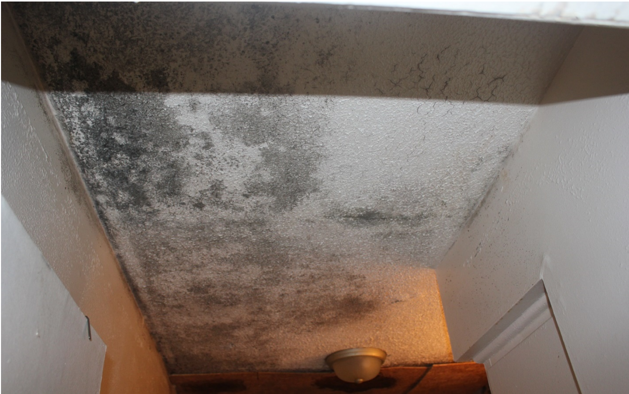
Bathroom hole in ceiling covered by a piece of plywood and mold growth across the ceiling and making its way down the walls.
