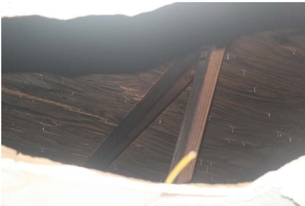
Kitchen ceiling is beginning to show signs of water damage.
