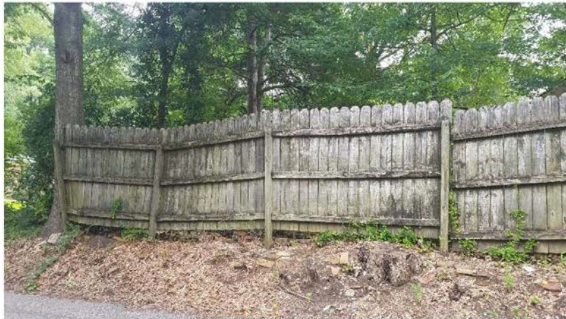
Figure 3: View of Corner of Fence on Ernest H. Jones Jr. Drive
