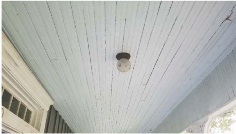
Figure 13: Existing Light Fixture
