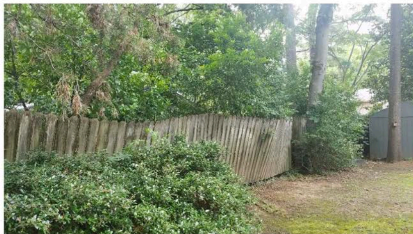
Figure 6: Buckling of Fence Along Property Line
