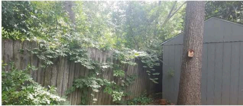
Figure 7: Buckling of Fence Along Neighboring Property
