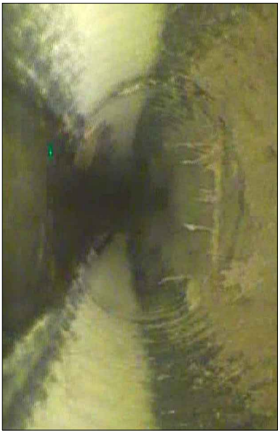
1 GAS LINE THRU PIPE (13' FROM INLET 2) C1.0
