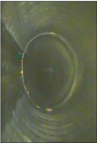
4 PIPE TO PIPE CONNECTION (113' FROM INLET 1) C1.0
