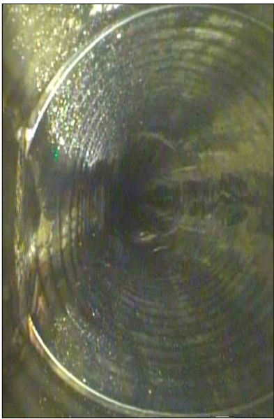
7 PIPE TO PIPE CONNECTION (42' FROM INLET 1) C1.0
