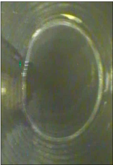
3 PIPE TO PIPE CONNECTION (133' FROM INLET 1) C1.0
