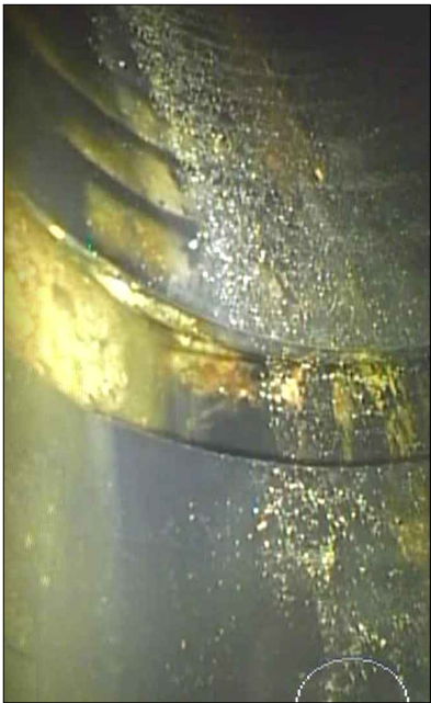
9 PIPE TO PIPE CONNECTION (10' FROM INLET 1) C1.0
