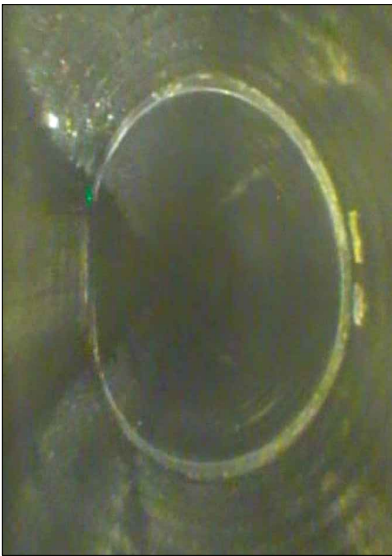
5 PIPE TO PIPE CONNECTION (94' FROM INLET 1) C1.0
