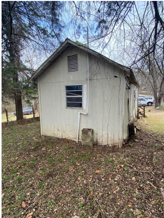
South side of structure
