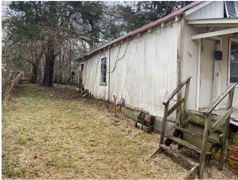
East Side of structure
