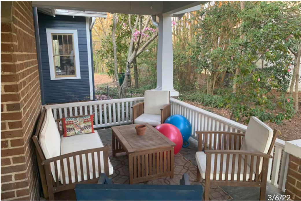
Front Porch (facing North)
