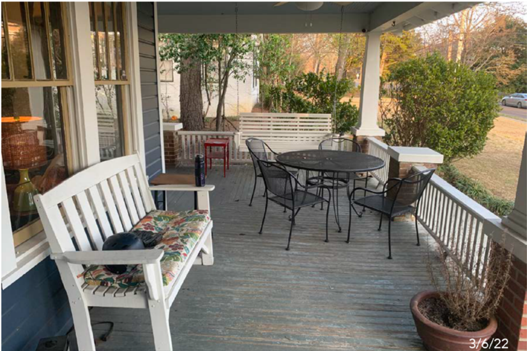
Front Porch (facing East)
