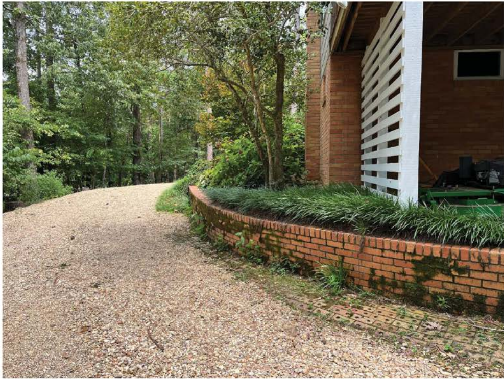
Figure 2. The northwest corner of 227 Lakewood. Note the pre-existing retaining wall. This wall and its retained soil should remain for structural reasons.
