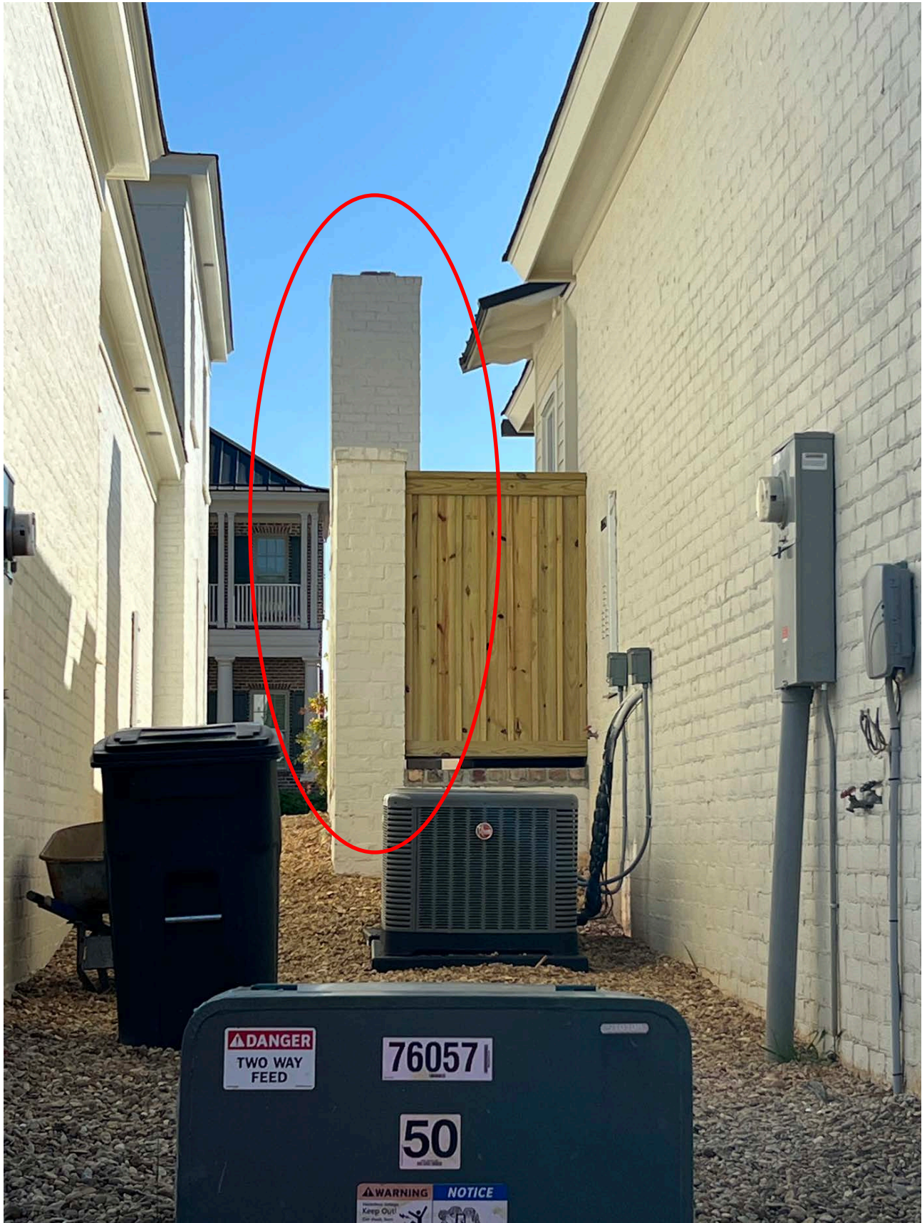
Attachment 4- View of fireplace from alley looking south
