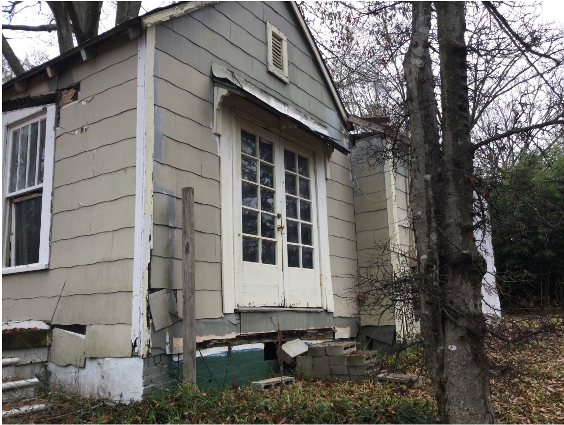
(RIGHT SIDE OF PROPERTY SOUTH SIDE OF THE PROPERTY)
