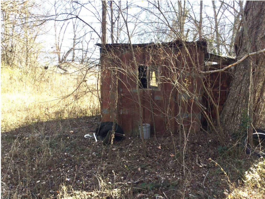
(LEFT SIDE OF STRUCTURE)
