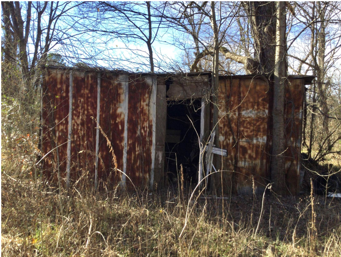
(BACK OF STRUCTURE)
