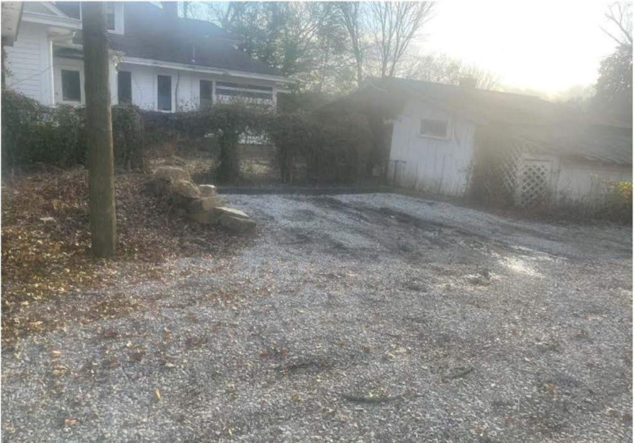
Exhibit 2. Current condition after work performed in November 2022.
