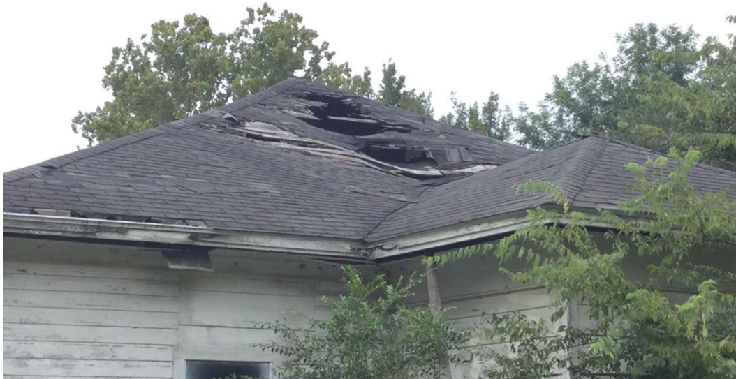
(WEST SIDE OF PROPERTY)
