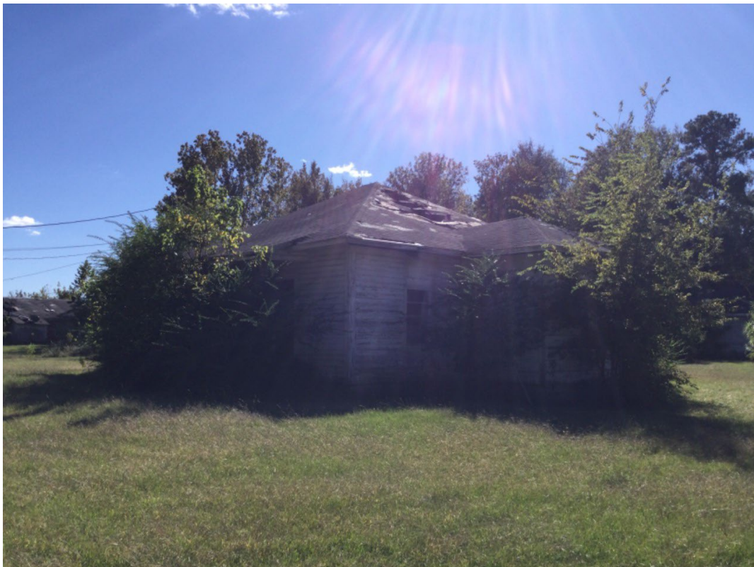
(WEST SIDE OF PROPERTY)
