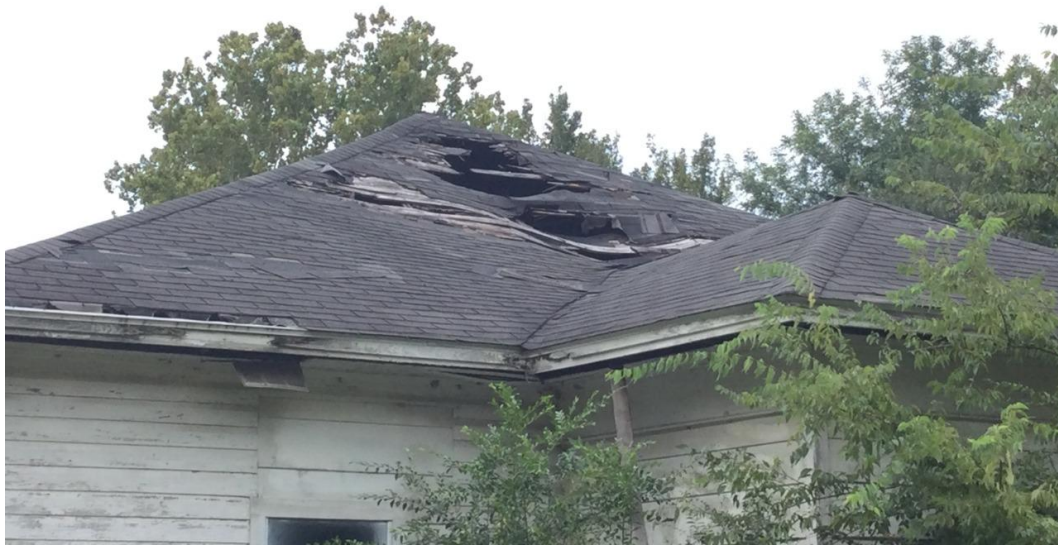
(WEST SIDE OF PROPERTY)
