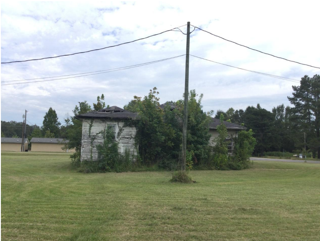
(SOUTH SIDE OF PROPERTY)
