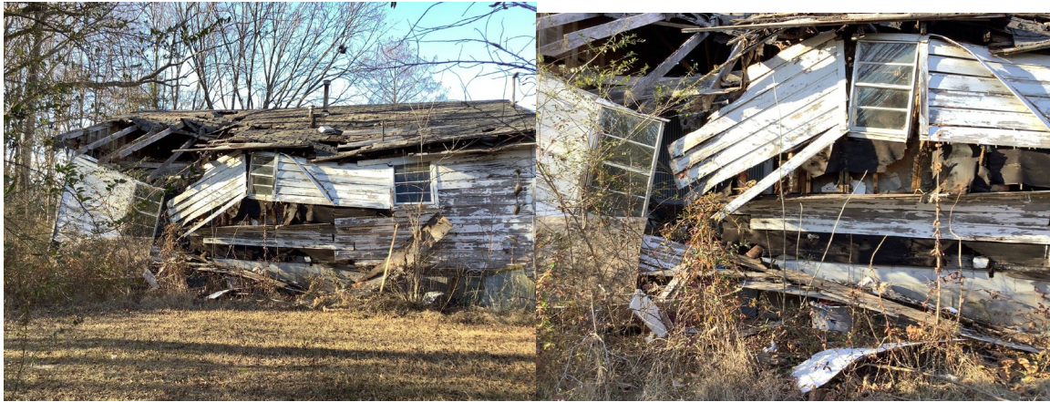
(SOUTH SIDE OF PROPERTY)
