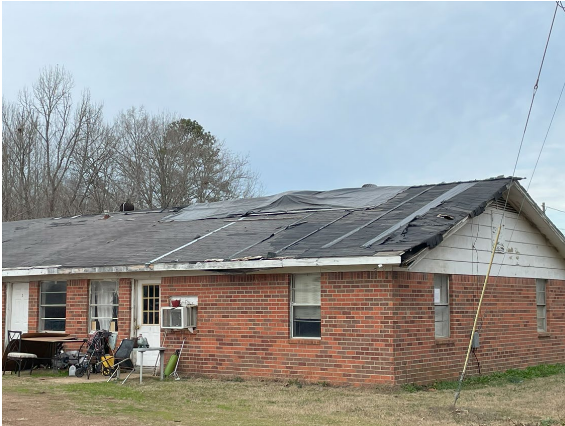
(EAST SIDE OF THE STRUCTURE)
