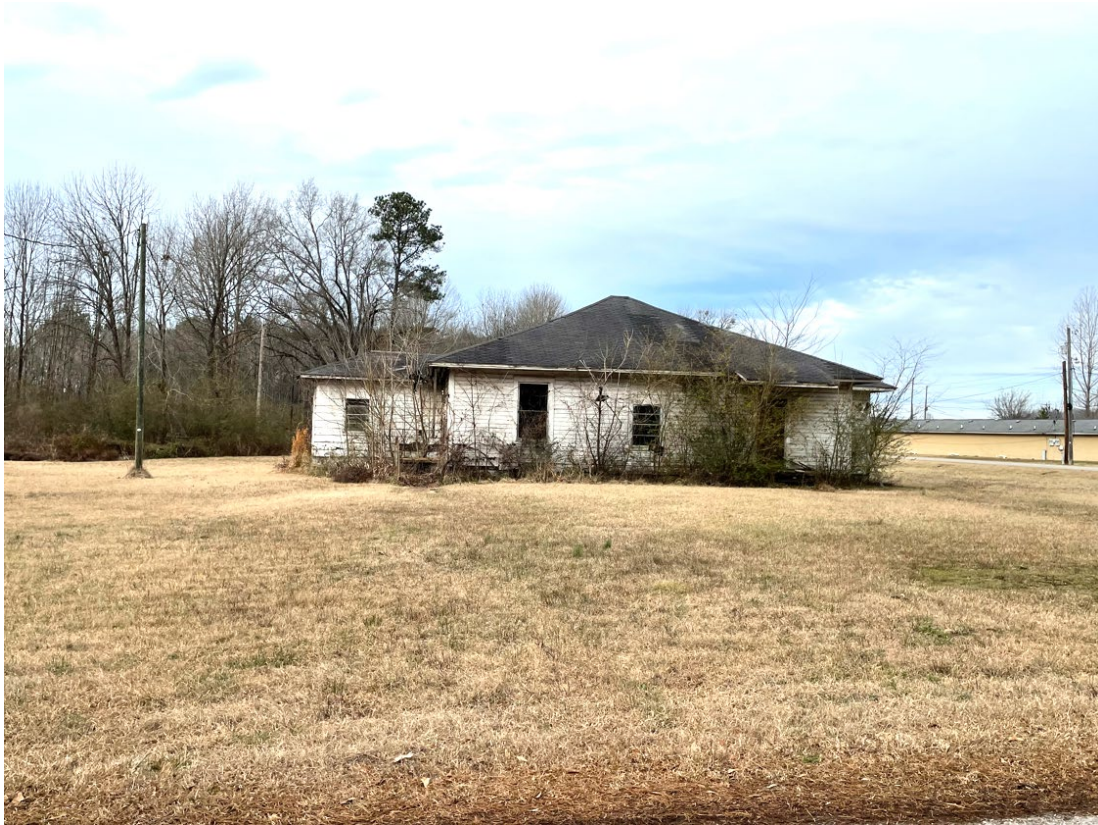
(EAST SIDE OF THE STRUCTURE)
