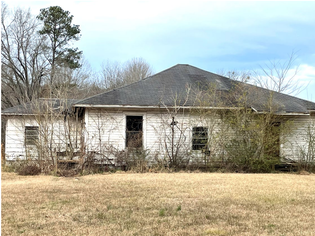
(SOUTH SIDE OF THE STRUCTURE)
