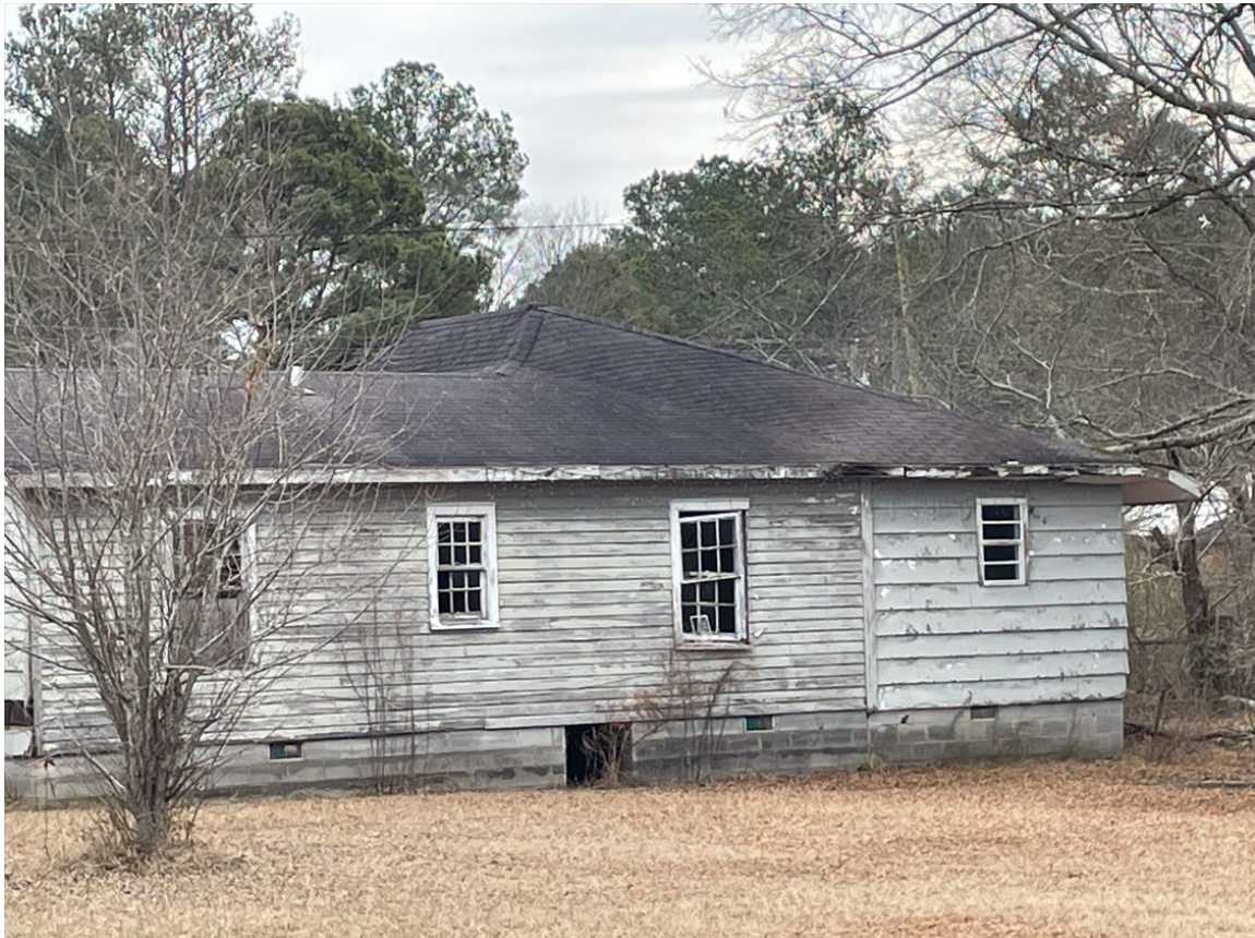
(EAST SIDE OF THE STRUCTURE)
