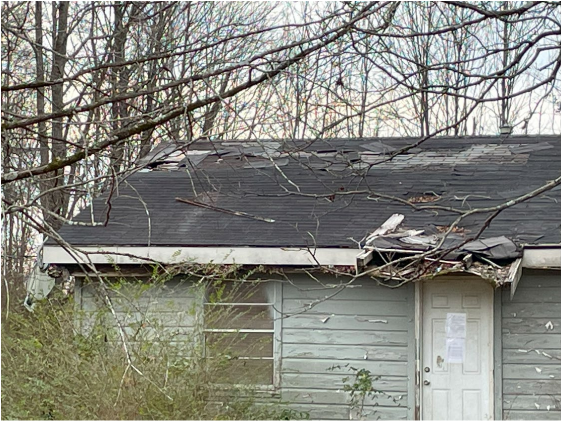
(EAST SIDE OF THE STRUCTURE)
