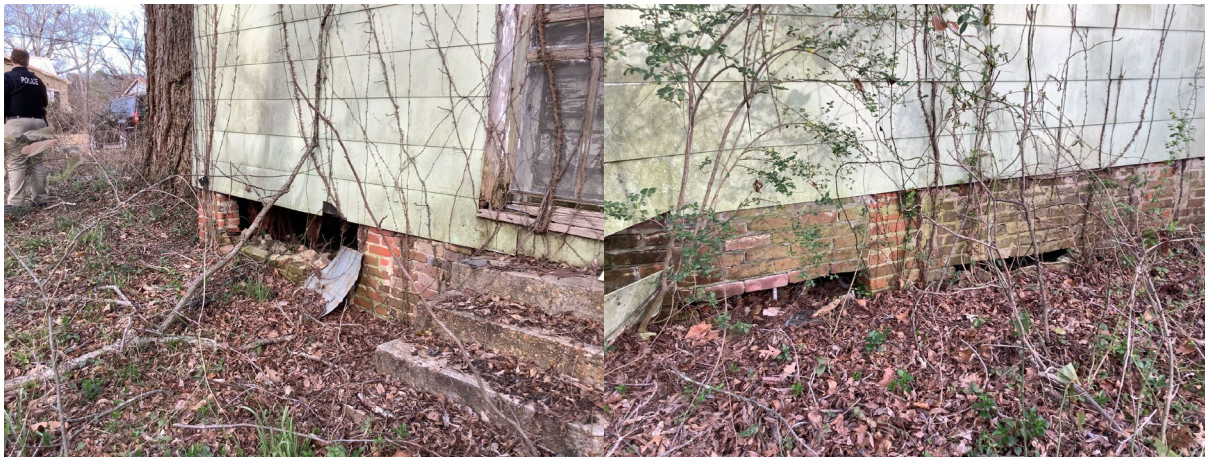
(SOUTH SIDE OF PROPERTY)
