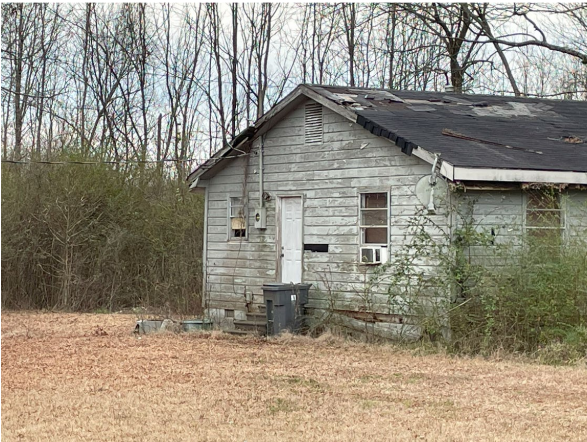
(SOUTH SIDE OF THE STRUCTURE)
