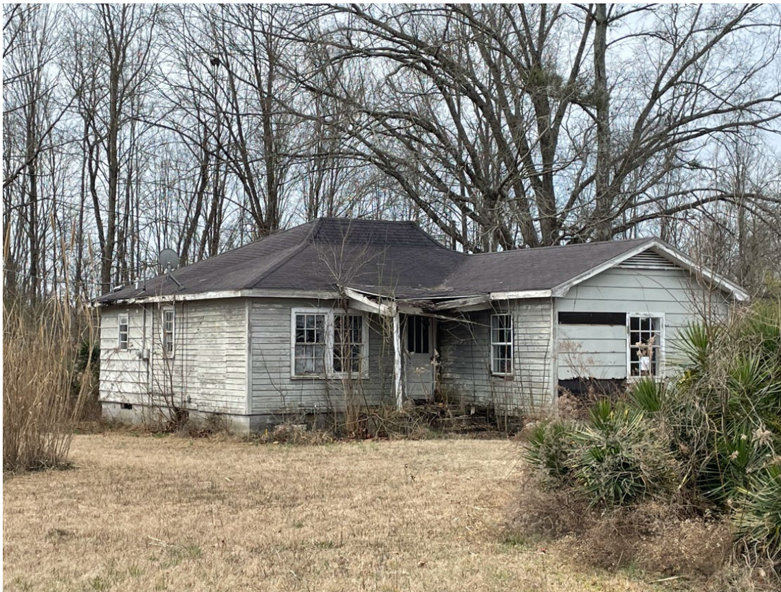
(WEST SIDE OF THE STRUCTURE)
