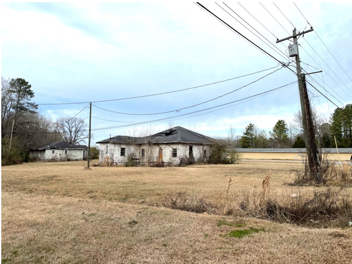
(WEST SIDE OF THE STRUCTURE)
