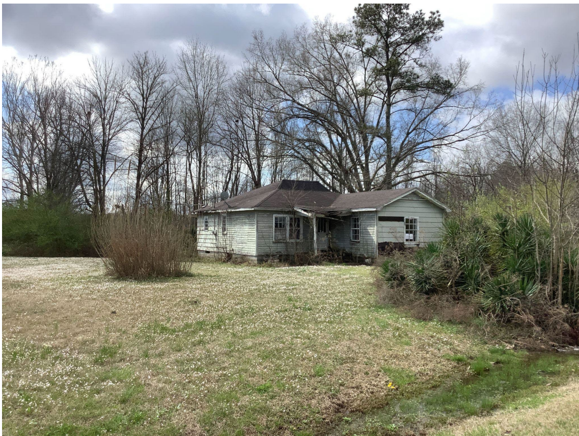
(EAST SIDE OF THE STRUCTURE)
