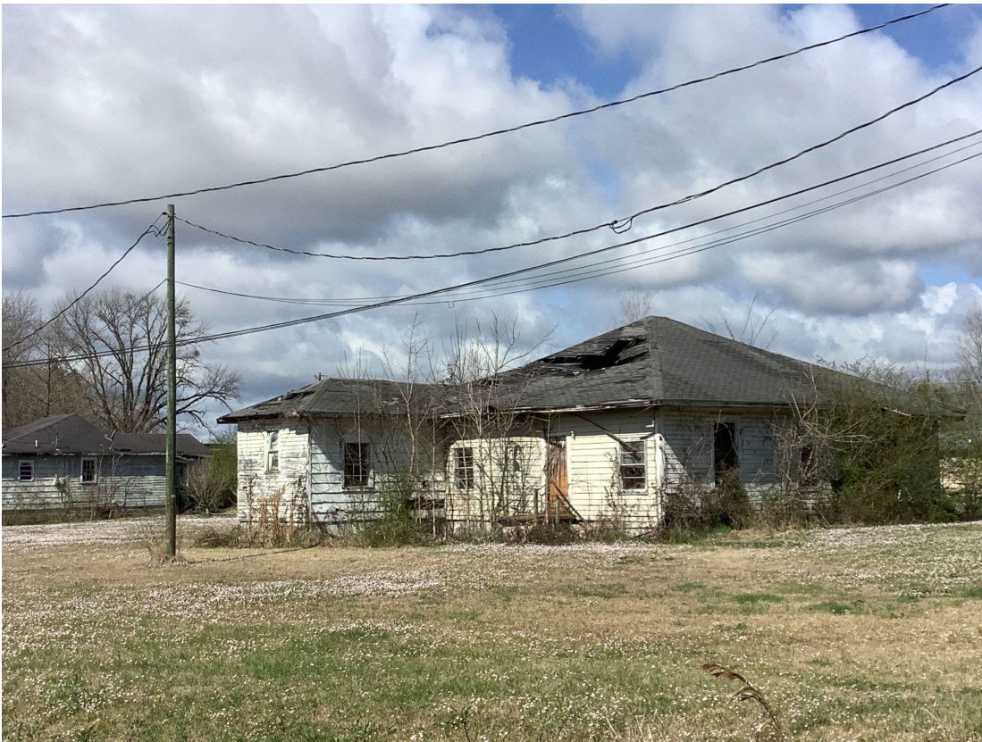
(WEST SIDE OF THE STRUCTURE)
