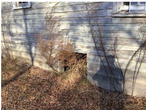
(SOUTH SIDE OF PROPERTY)
