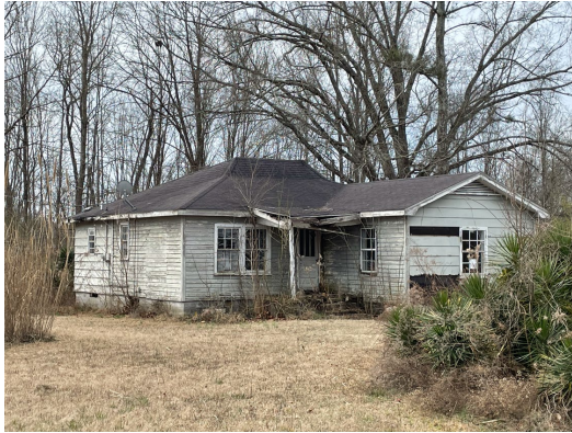
(WEST SIDE OF THE STRUCTURE)
