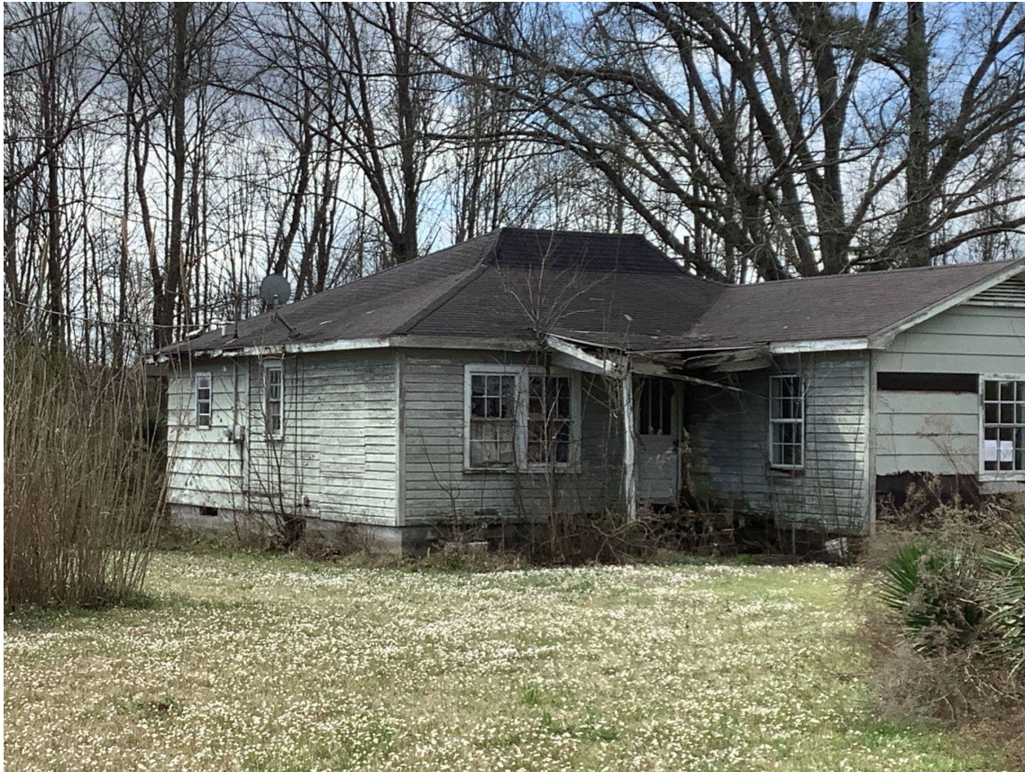
(NORTH EAST SIDE OF THE STRUCTURE)
