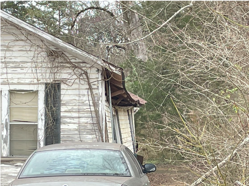
(WEST SIDE OF PROPERTY)
