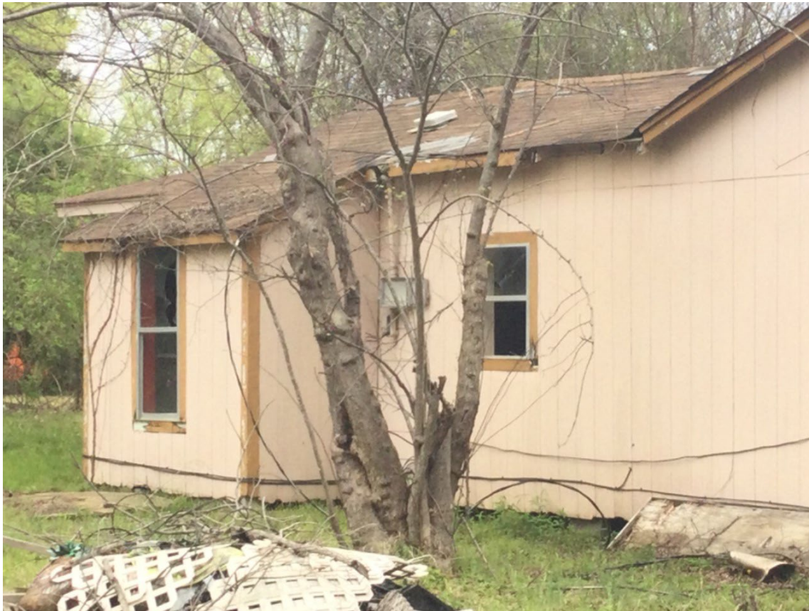
(SOUTHWEST CORNER OF THE STRUCTURE)
