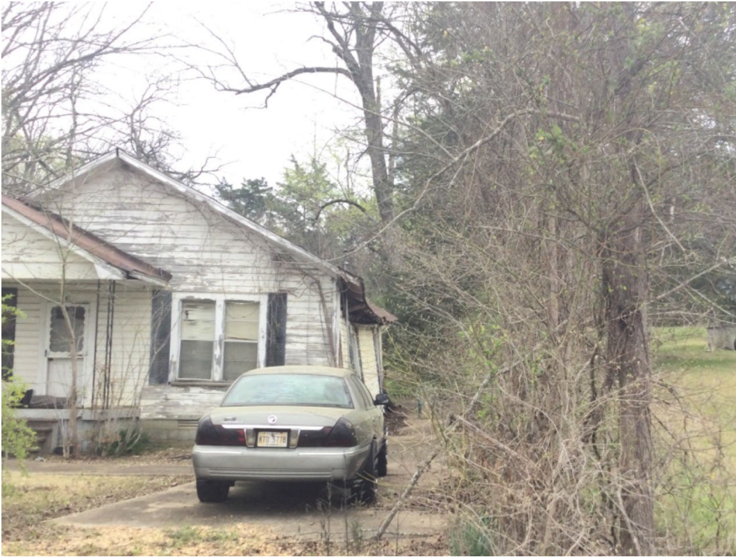
(WEST SIDE OF PROPERTY)
