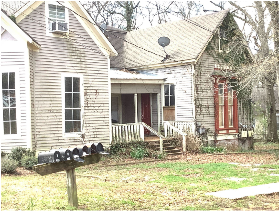
(SOUTH SIDE OF THE STRUCTURE)
