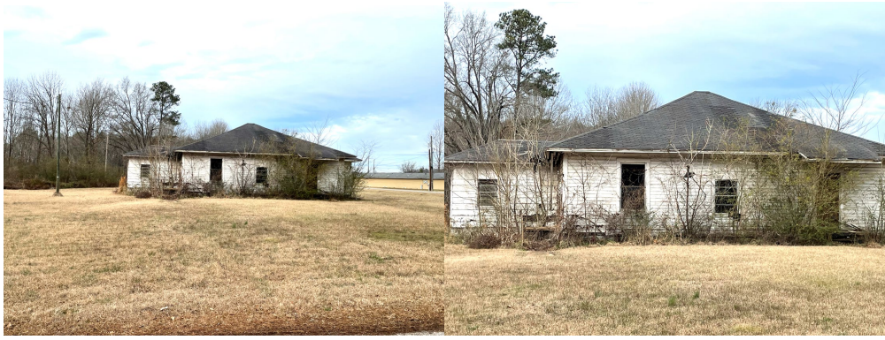
(SOUTH SIDE OF THE STRUCTURE)
