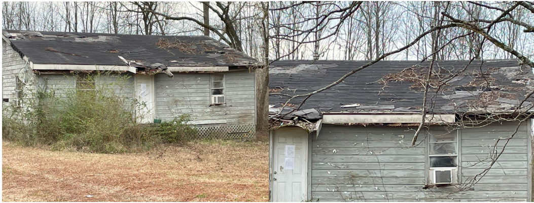
(EAST SIDE OF THE STRUCTURE)
