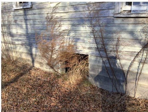
(SOUTH SIDE OF PROPERTY)
