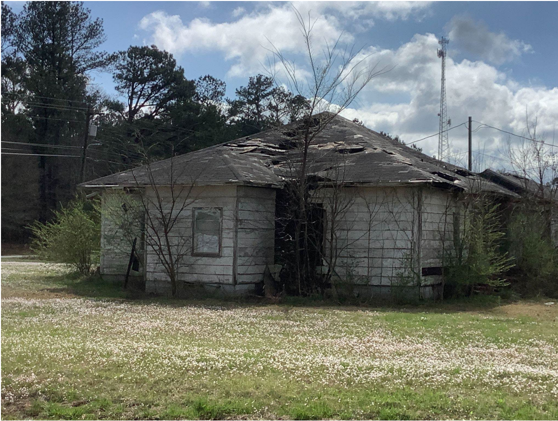
(SOUTH EAST SIDE OF THE STRUCTURE)
