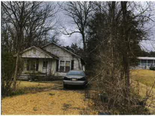
(WEST SIDE OF PROPERTY)
