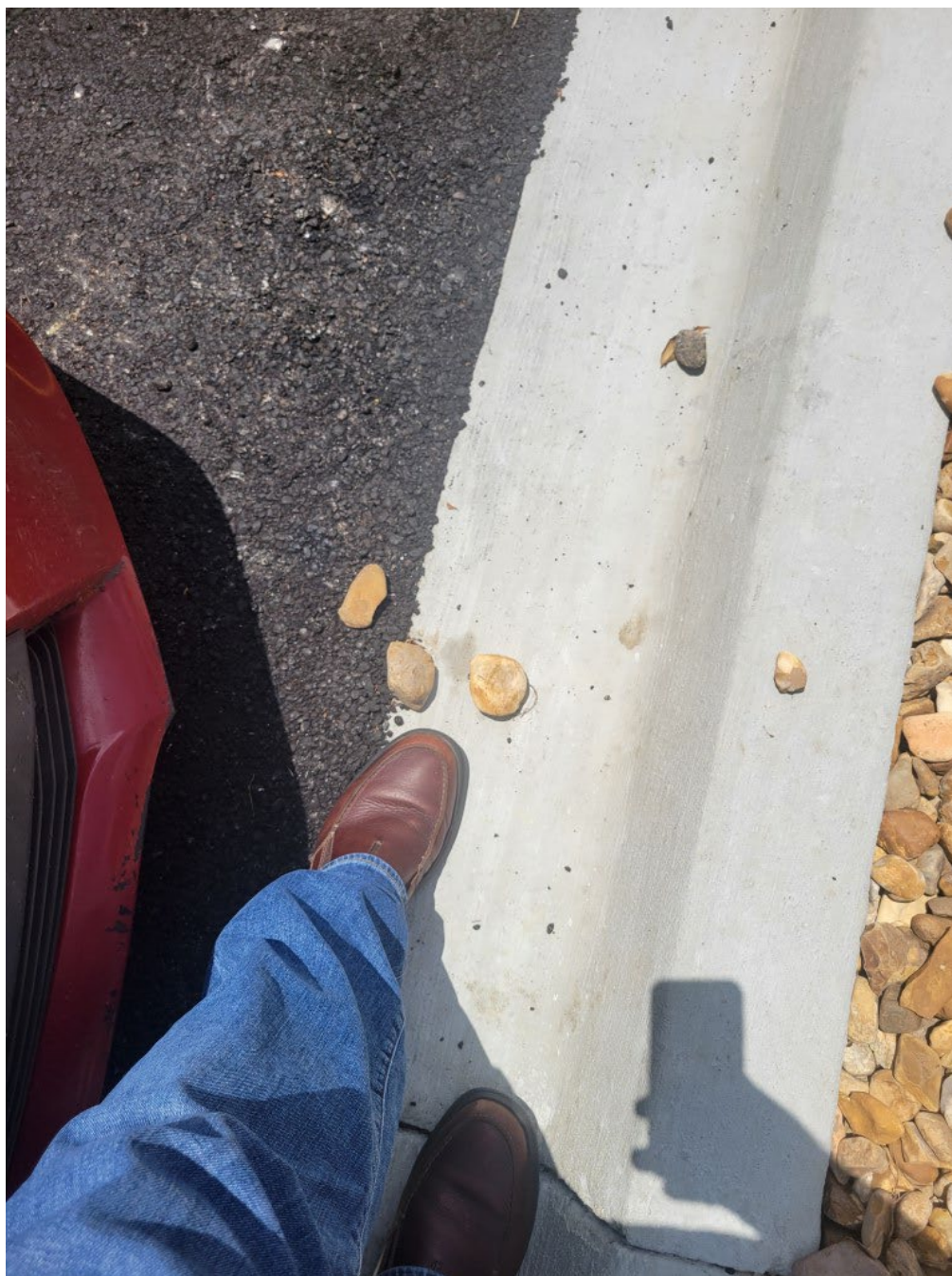
Rocks present a tripping hazard
