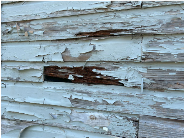
The outside of the structure
