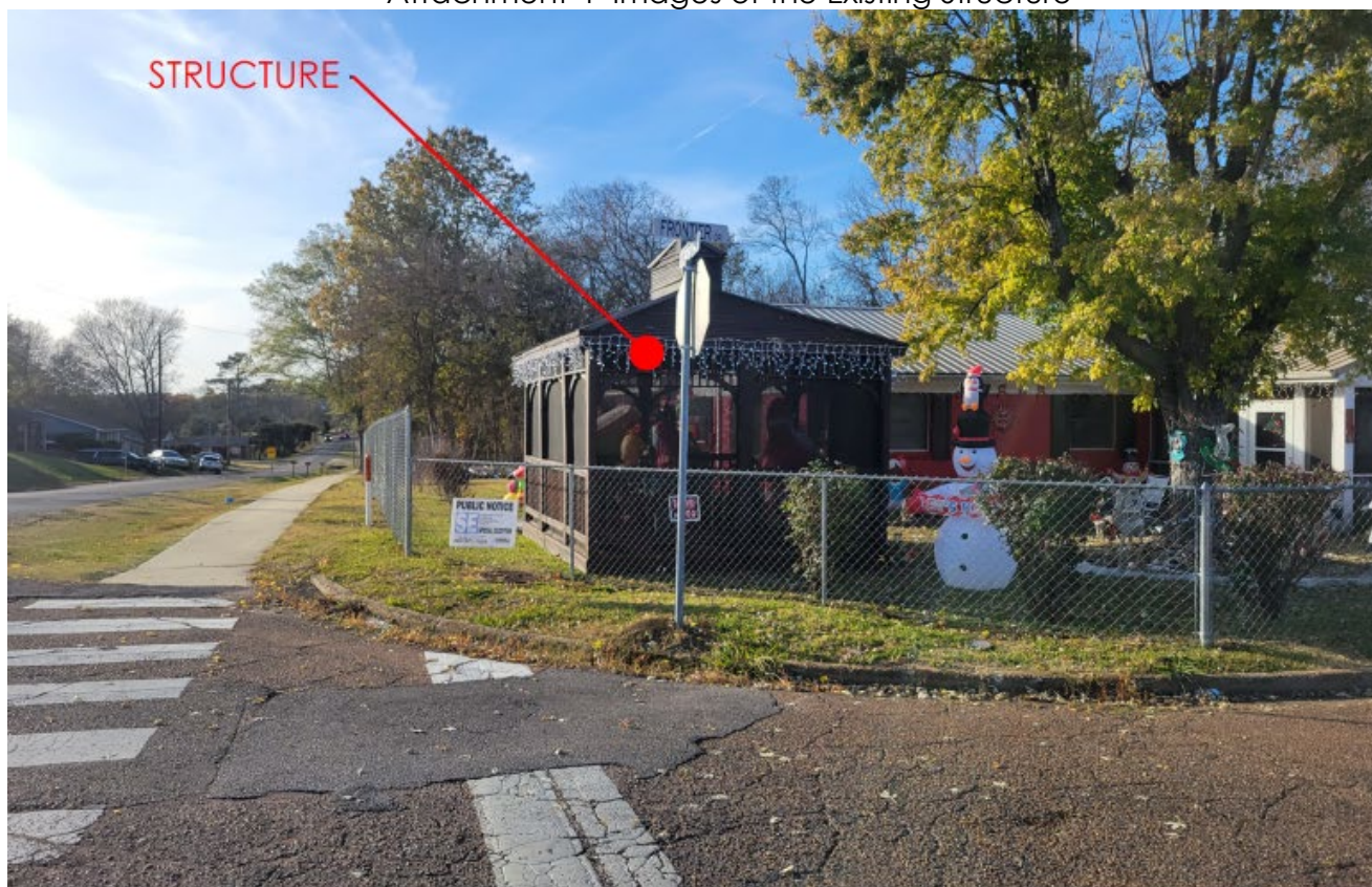
Attachment 4- Images of the Existing Structure
