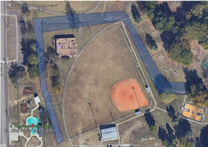
J.L. King Sr Memorial Park stream buffer zone and post-construction zone
