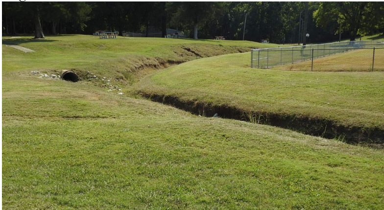
Rilling, channel erosion and sedimentation at JL King Park drain swale
