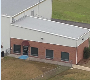
Aerial View of Current FBO
