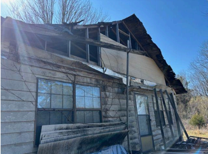
Bracing holding up walls from giving away.
