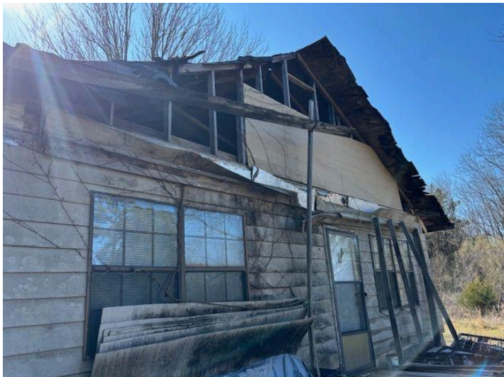
Bracing holding up walls from giving away.
