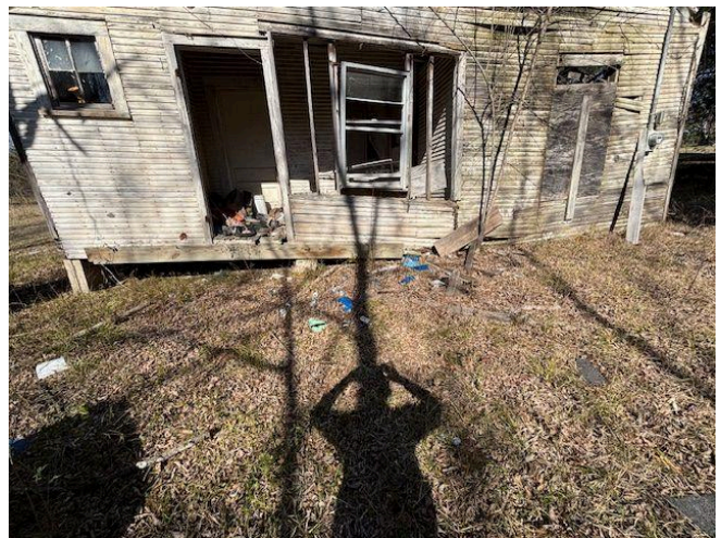
Rotten wood unsafe for front porch entry
