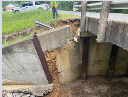
WINGWALL FAILURE
