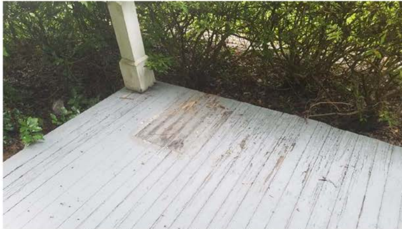
Figure 9: Detail of Existing Porch Floorboard Repair
