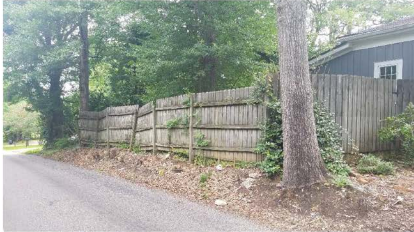
Figure 2: View of Fence from Ernest H. Jones Jr. Drive
