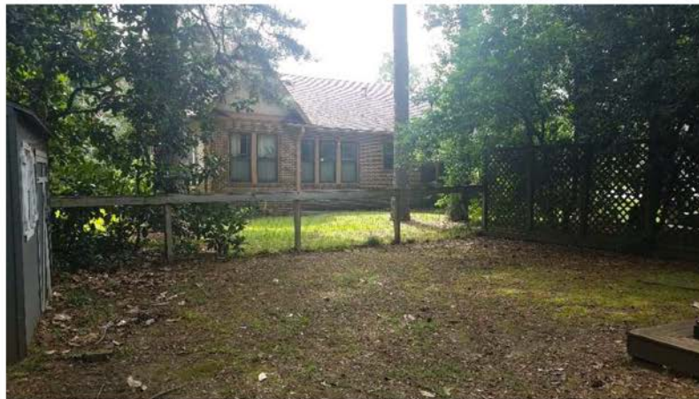
Figure 8: Small Wire Fence Along Property Line with 408 Greensboro Street, With Trellis Fence Visible
