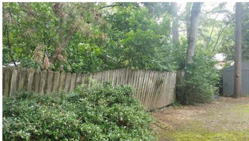
Figure 6: Buckling of Fence Along Property Line
