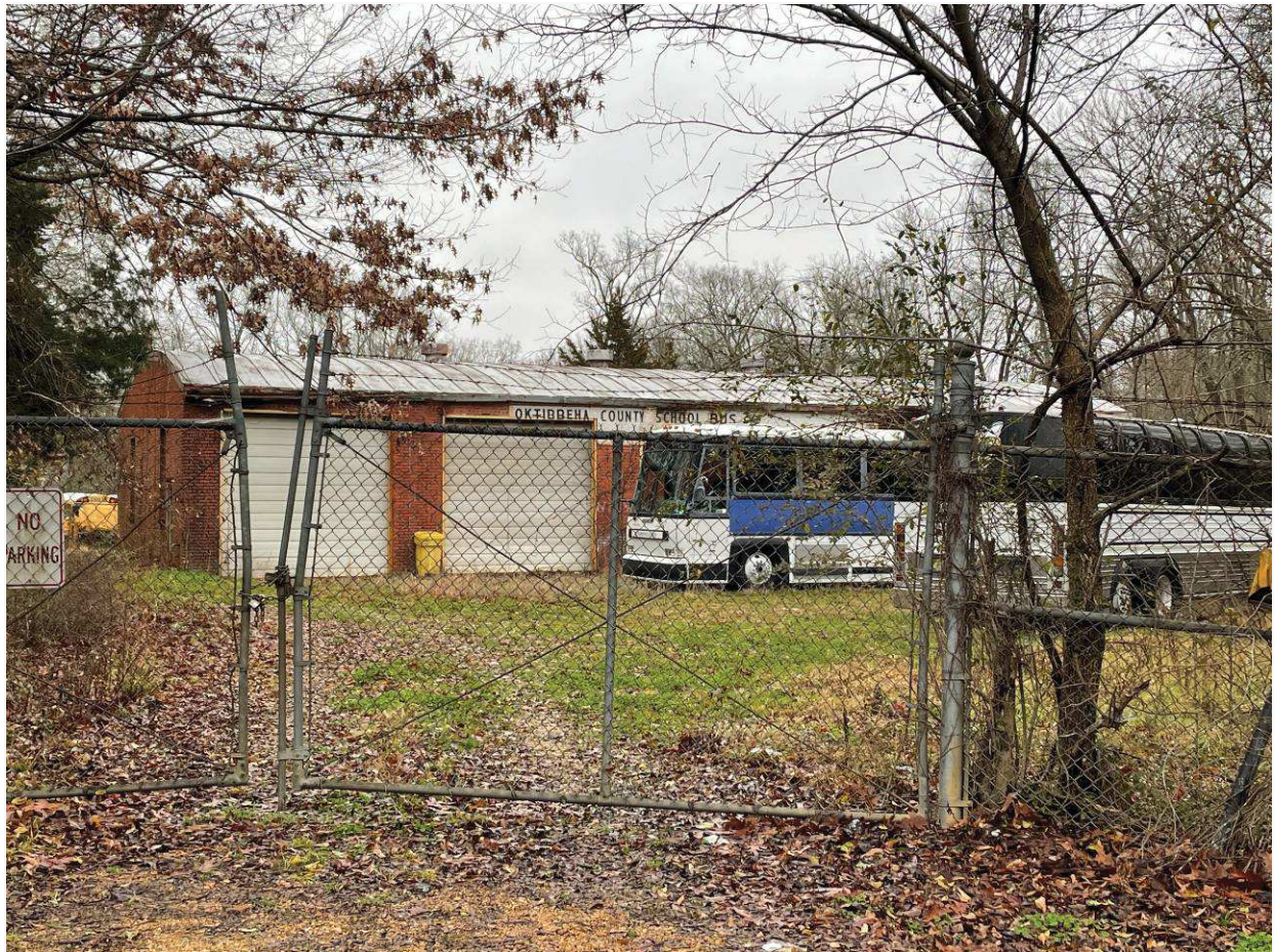
Figure 21: Oktibbeha County School Bus Shop. 220 Gillespie Street, West. J Rosenberg, Feb. 4, 2022
