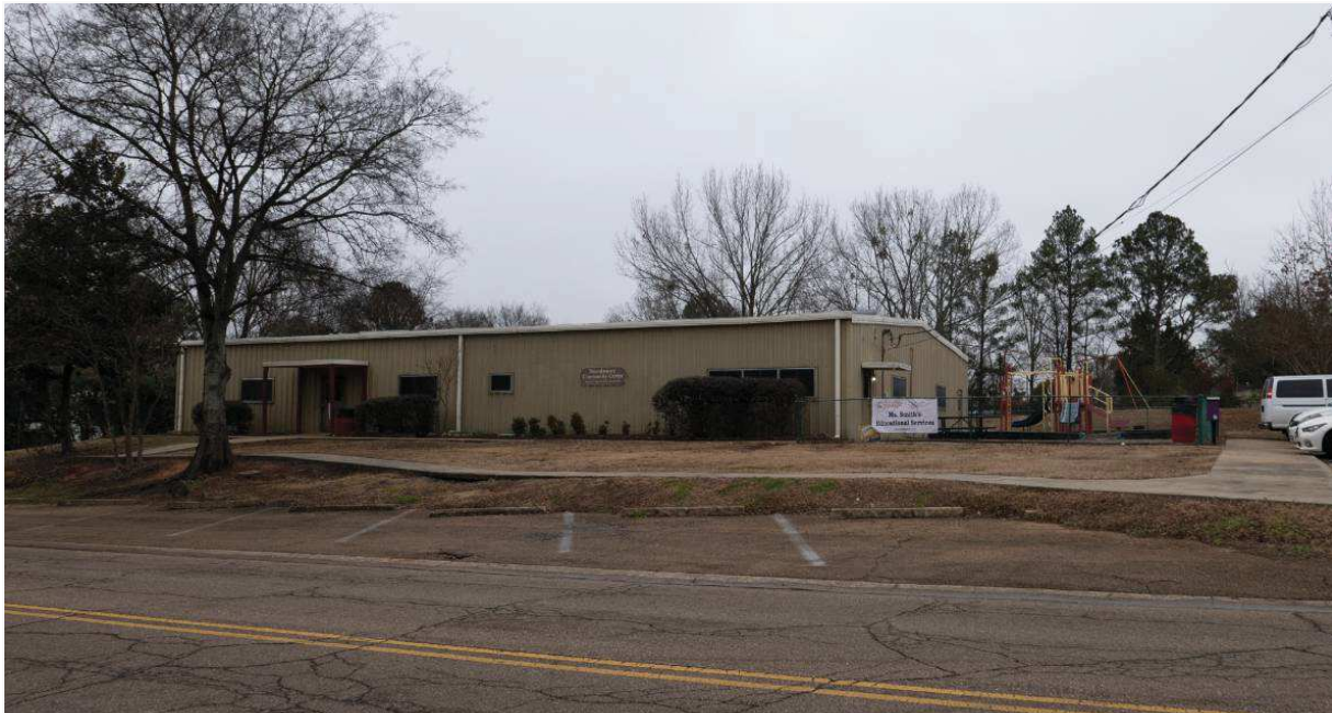
Figure 28: Needmore Community Center. 610 Gillespie Street East. J Rosenberg, Feb. 4, 2022
