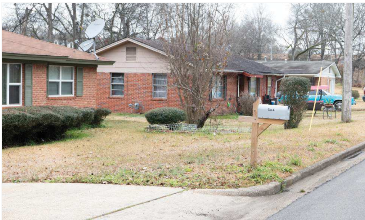
Figure 14: 500 block Hancock Street, looking north. J Rosenberg, Feb. 4, 2022
